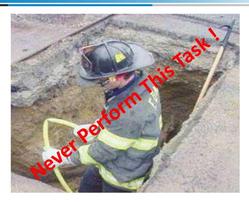
A firefighter easily bends this plastic pipe, but doing so could result in a static spark that ignites leaking gas. "Do not approach or touch leaking plastic pipe" or operate any Gas Valves. Wait for the Utility!
