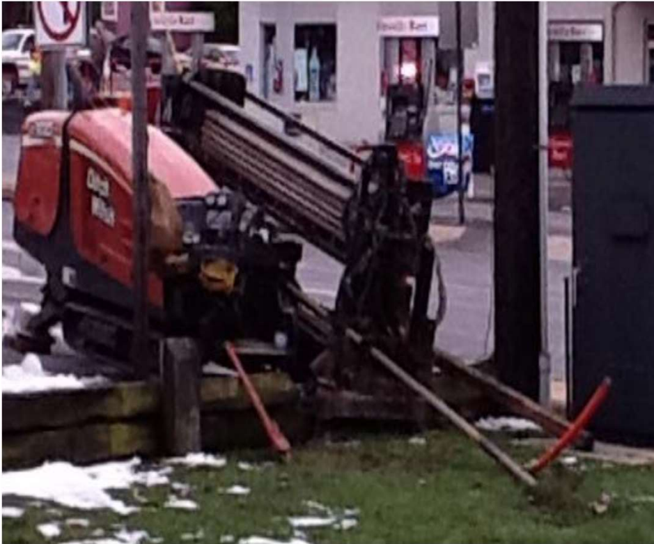
Horizontal Directional Drilling
